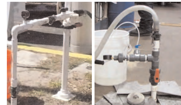
Typical well head assemblies for delivery of VeruSOLVE-HP™
