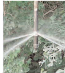
Typical In-Situ application by geoprobe
