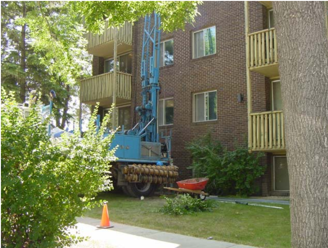
FIGURE 4. The corner of the apartment building that the soil beneath it is contaminated with benzene and other hydrocarbon compounds. The rig is drilling a well less than one metre from the side of the building where an electrode will be subsequently located.
